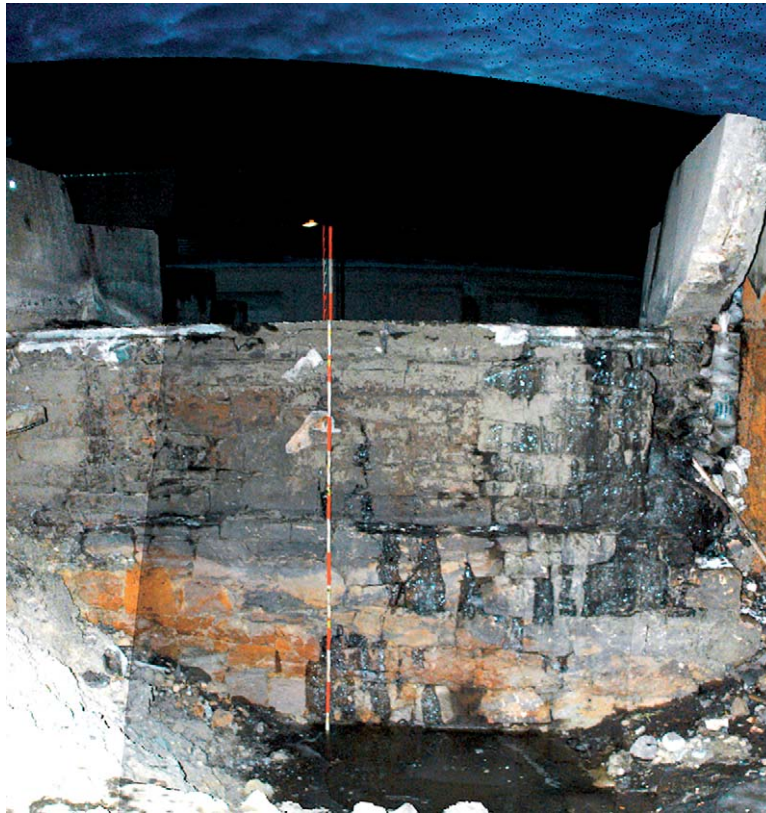
Figure 10 2003–04/Stanhope, New Jersey. Overlapping digital photo composite of the visible color channel (what the LIDAR ‘saw’) of the exposed eastern face of the 1830-era Furnace Falls Dam, produced by a Nikon digital camera computer synchronized with the Riegl LIDAR scan. Each color pixel was matched, pixel by pixel, to the 6 mm-precise, LIDAR scanner-derived, coordinate points – rendering the true color, 3D data captures of the formerly submerged dam. Temperature range during this operation: 10–14° F. © 2007 Joel W. Grossman, PhD. Published by Elsevier Inc. All rights reserved.
