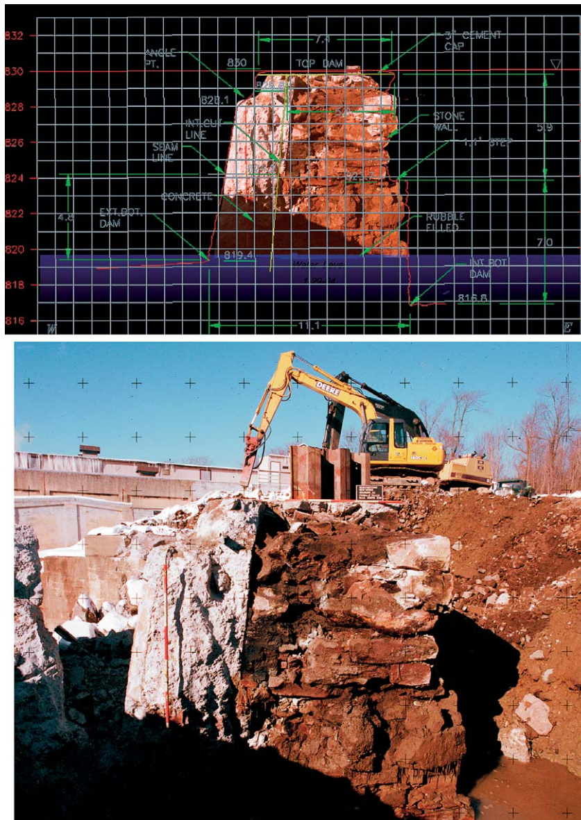
Figure 13 2003–04/Stanhope, New Jersey. (Bottom) Metric photo of sectioned historic dam profile, captured with Rolleimetric camera as the historic dam was sectioned and impounded river water was released to unblock the flood-damaged channel. Note the imbedded calibration marks used to correlate metric photograph with real-world coordinates recorded by the laser-radar. (Top) Digital composite of Rolleimetric photo of cross-section of 1830-era cut-stone dam – the metric photo is scaled, overlaid, and geo-referenced to LIDAR-derived elevation and dimension profile measurements. © 2007 Joel W. Grossman, PhD. Published by Elsevier Inc. All rights reserved.
